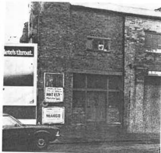
This narrow little building at 180 Bradford St., Birmingham, was the Jurek shop. It has now been demolished, following considerable disagreement with the U.K.'s Inland Revenue, and the machines and inventory sold off and, in short, Jurek makes pistols no more.
